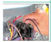
Attach the flagged end of the black wire to the Compressor Common on the "T" side of the contactor.
