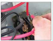
3] Remove the compressor Run wire from the contactor or Run Capacitor terminal, as applicable.
