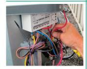
Remove the loose wire (from Step 7) from the active input of the contactor and attach the stripped end of the Active wire in its place.
