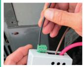
Attach the black wire(supplied) to Compressor Common on the SureStart green terminal connector.
