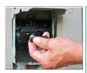
Turn off all power to the HVAC unit at the circuit breaker..
