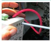
Attach the compressor Run wire to the SureStart Run Winding terminal.
