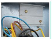
Secure the mounting bracket for the SureStart inside the control
