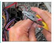
Strip the compressor Run wire a least 1/2 in.\* Crimp appropriate size Ferrule (supplied) onto it.
