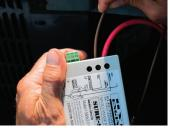
Attach the brown wire supplied with the SureStart to the Run Capacitor terminal on the SureStart.
