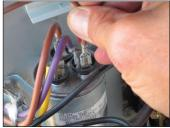
Identify the cable connecting the contactor and the Run Cap. Remove this connection to the Run Cap Attach the flagged end of the brown wire to the same terminal of the Run Cap#1.
